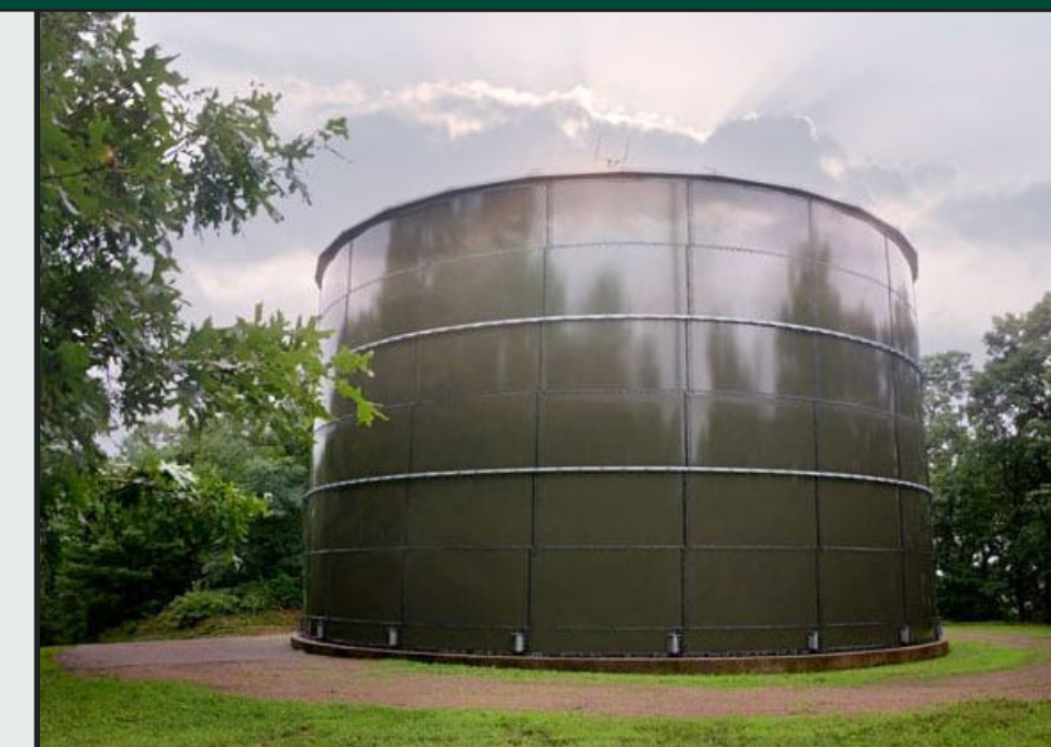
Glass Fused to Steel Bolted Reservoir
